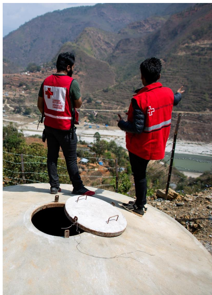
Water system newly constructed by the Nepalese Red Cross Society, in partnership with the IFRC, the Canadian Red Cross and the Danish Red Cross, in the remote earthquake-affected village of Kharelthok, Nepal ©Canadian Red Cross, Marko Kokic, March 2017
